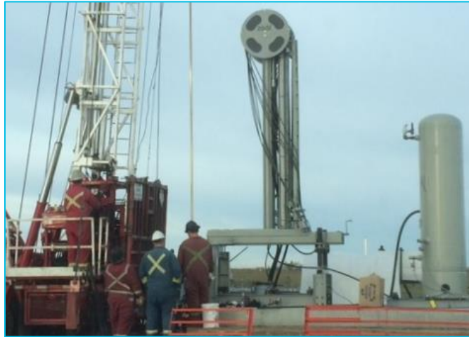
Lift System secured at middle of support structure during workover
